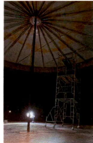
Well site 3-350K water storage tank rehab project
